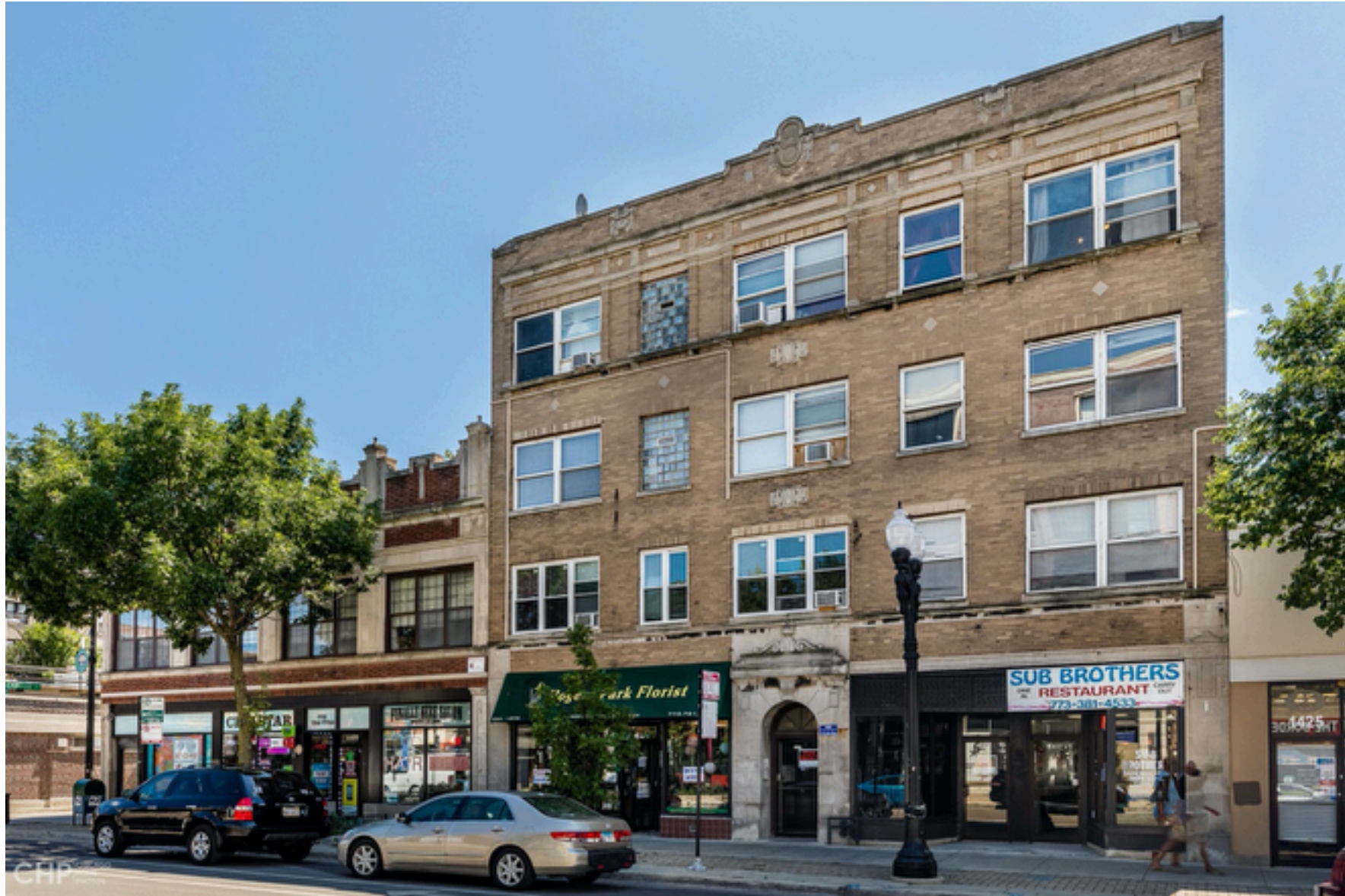
Front View of Existing Building
