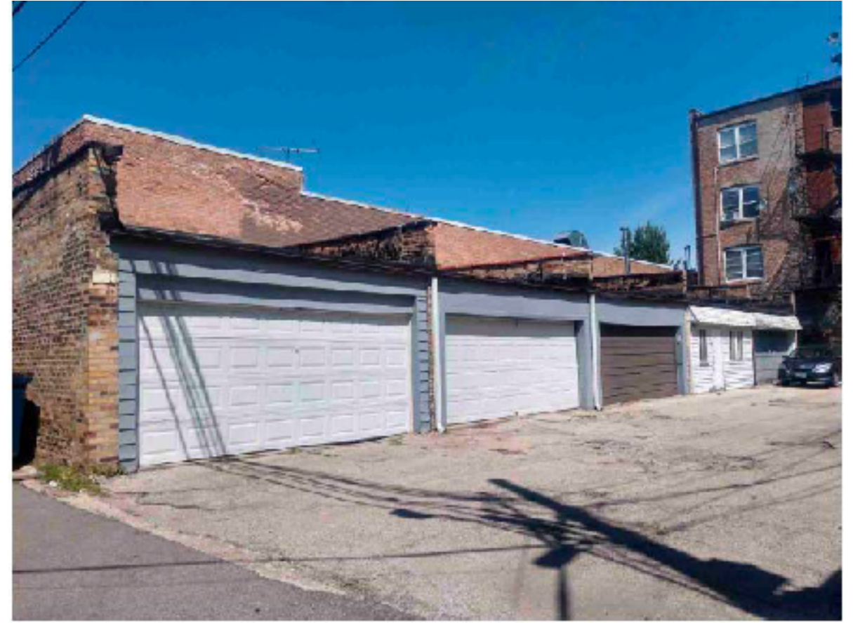
Alley View of Existing Conditions
