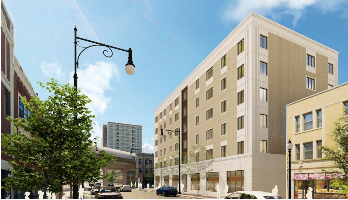
Phase I – East View Howard St
